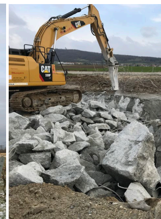
Recycling old foundations at Berg repowering
